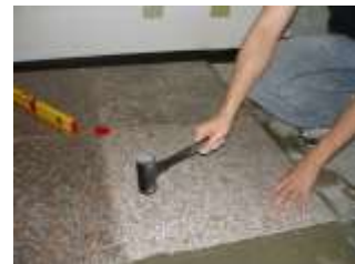
insert tile spacers, form 3 mm gap for grouting, check leveling
