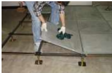
Install access panel and check level in sequence
