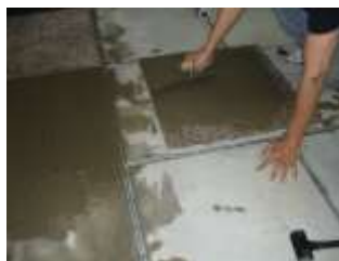
apply adhesives on tiles
