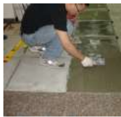
apply adhesive on panels
