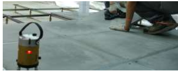
Install access panel and check level in sequence
