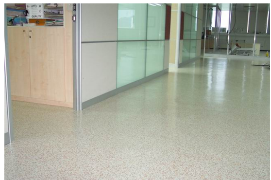
Actile to install on low-profile access floor (with cable trenches) after cable routing
