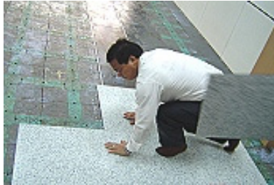
install Actile on existing access floor
