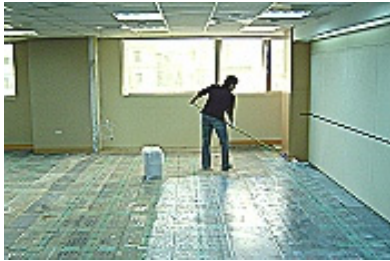
remove old carpet tiles brushing releasable adhesive
