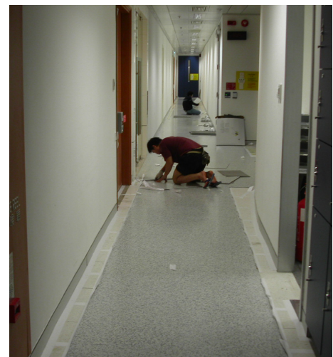
retrofitting on old HPL access floor, using double-side tape
