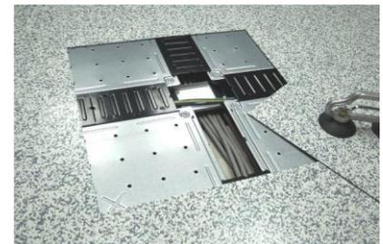
Remove first-piece tile by using one-cup or two-cup access floor lifter
