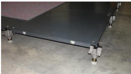
(4) Continuous installation at field
