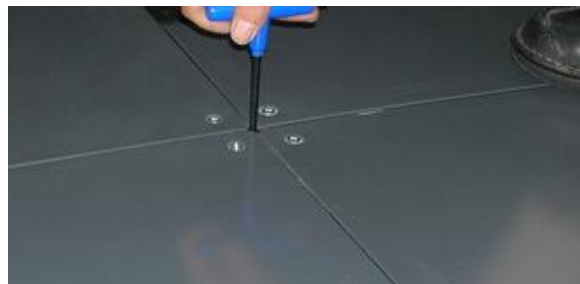
(5) 5 mm hexagon key wrench for height-adjustment and final check-up, clockwise upward, counter-clockwise downward. Turn pedestal until feeling gently grounding at the sub-floor.
