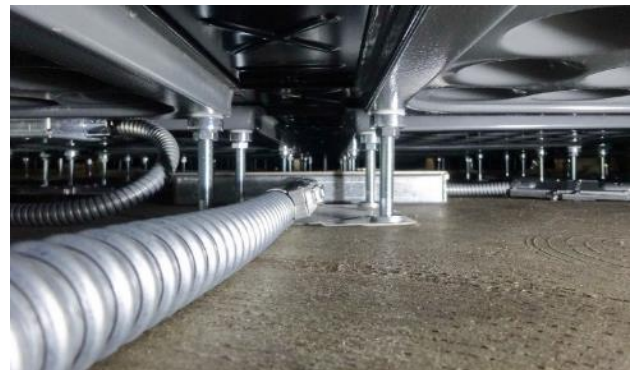
Jumpers connect zone boxes, floor boxes, and boxes under access floor.
